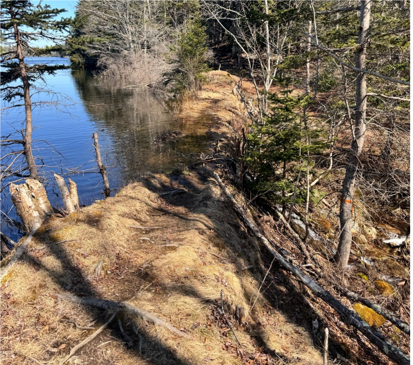
^ Looking along the 180ft ridge of the earthen dam at Lily Pond from the spillway following the March heavy rainfall event. There had been no previous evidence of overtopping at this spot.
