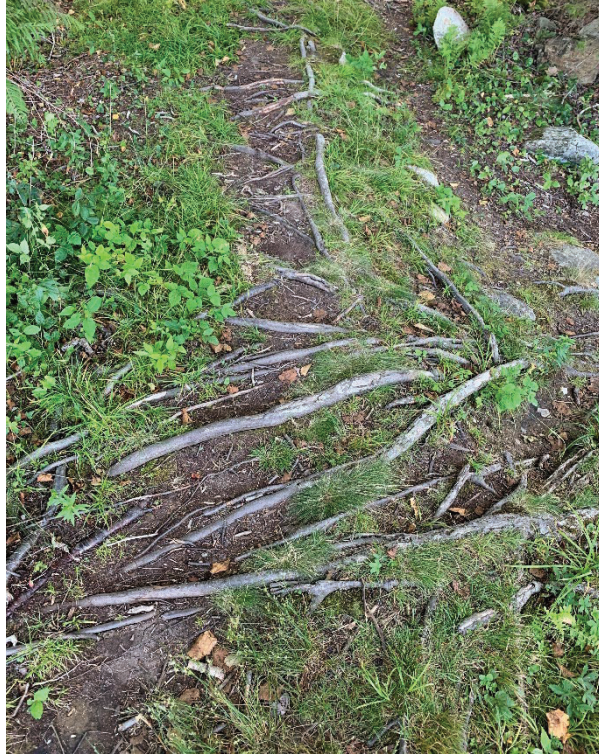
Photo 5.1: Woody root intrusion, typical along the majority of the dam
