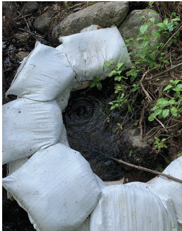
Photo 5.2: Significant hydraulic boil located along the dam toe adjacent to the Spillway
