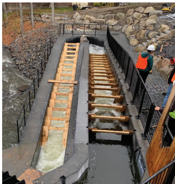
Example of a Denil fishway installed with two (2) ladder sections connected by a resting/turning pool
