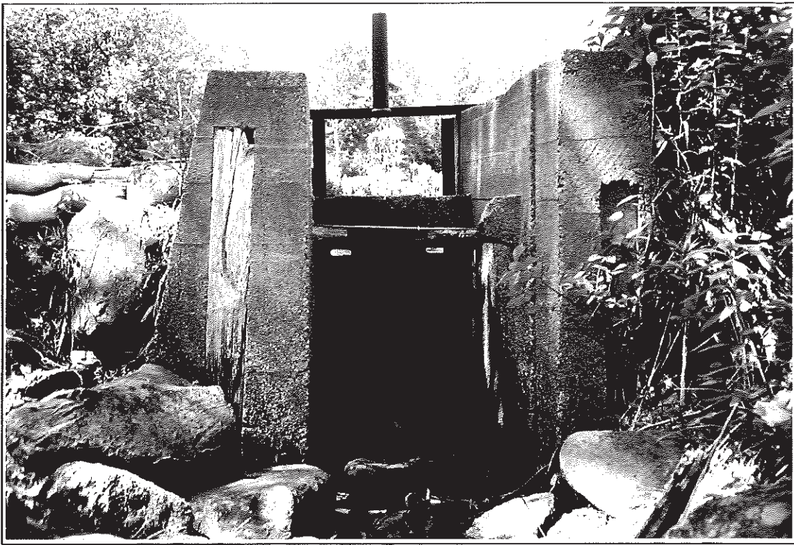
Photo B-1 Lily Pond Dam. Downstream View of Sluiceway Structure.
