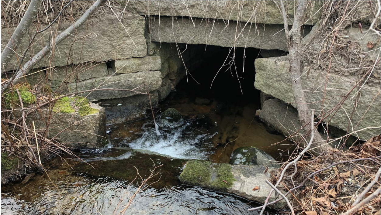
Route 15 Culvert Inlet - Looking Downstream
