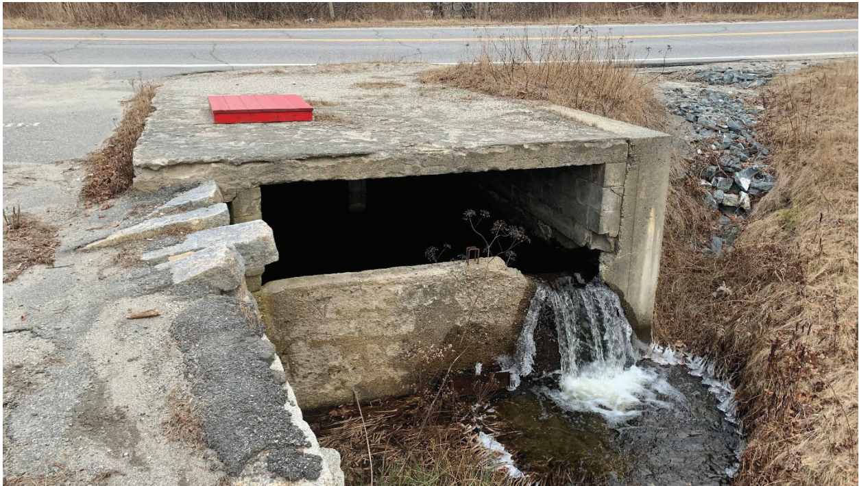
Fire Water Tank at Outlet of Culvert - Looking upstream with Route 15 in the Background
