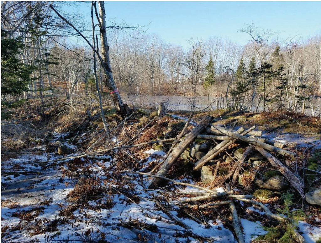
Tree removal from the dam in 2016
