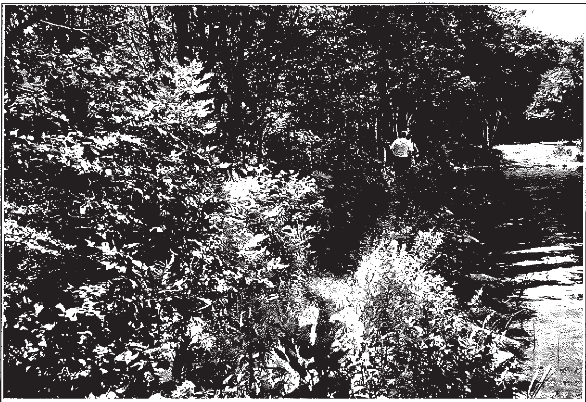
Photo B-4 Lily Pond Dam. Top and Upstream Slope of West Earthen Dike.
