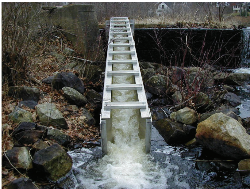
Example of an Alaska Steppass fishway installed at a Low-head Concrete Dam Image Credit: Sheepscot Fishways
