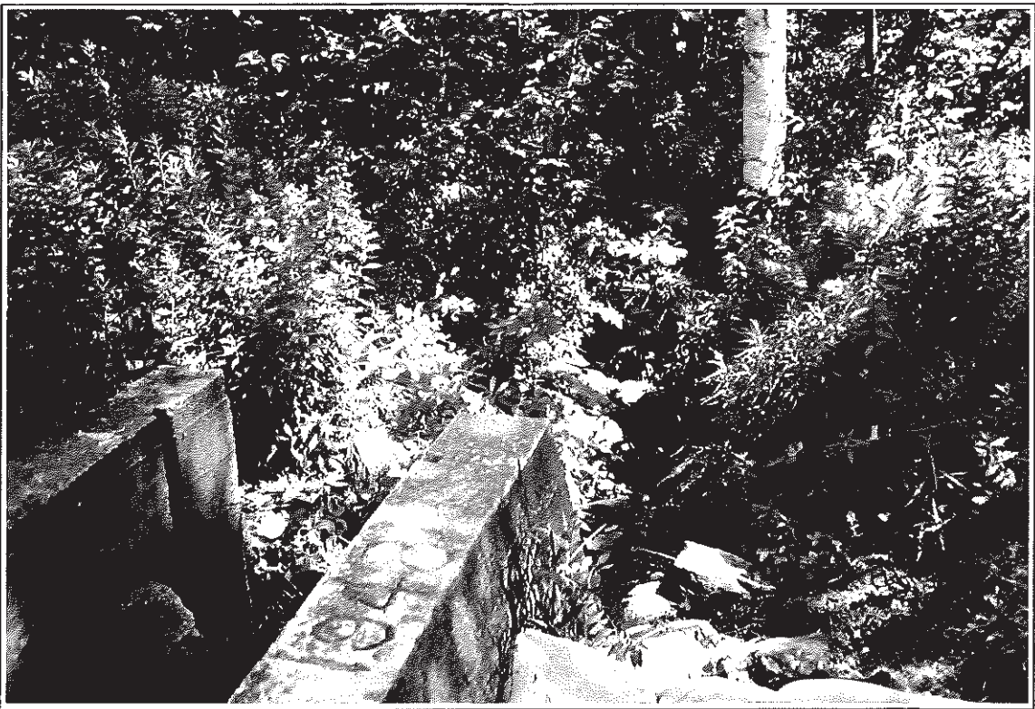
Photo B-2 Lily Pond Dam. Sluiceway and Downstream Channel.
