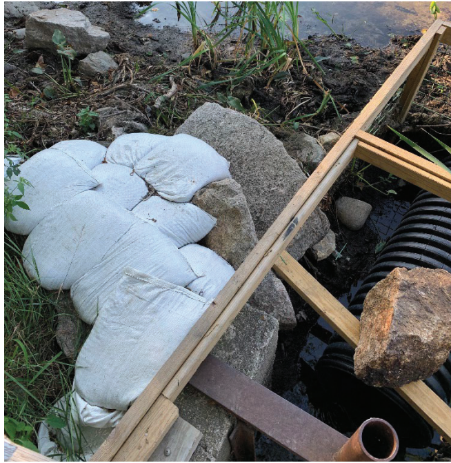
Photo 4.3: Area of Sandbag Reinforcement of Dam Embankment Erosion
