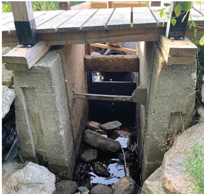
Photo 4.2: Two Foot (2’) Wide Concrete Spillway Structure with Metal Gate (8/8/2020)
